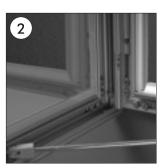
• Take out the metal bars from the slots inside the cover. Fix the cover in open position by leaning the ends of the metal bars to the plastic holder in the bottom and upper profiles of the frame.
